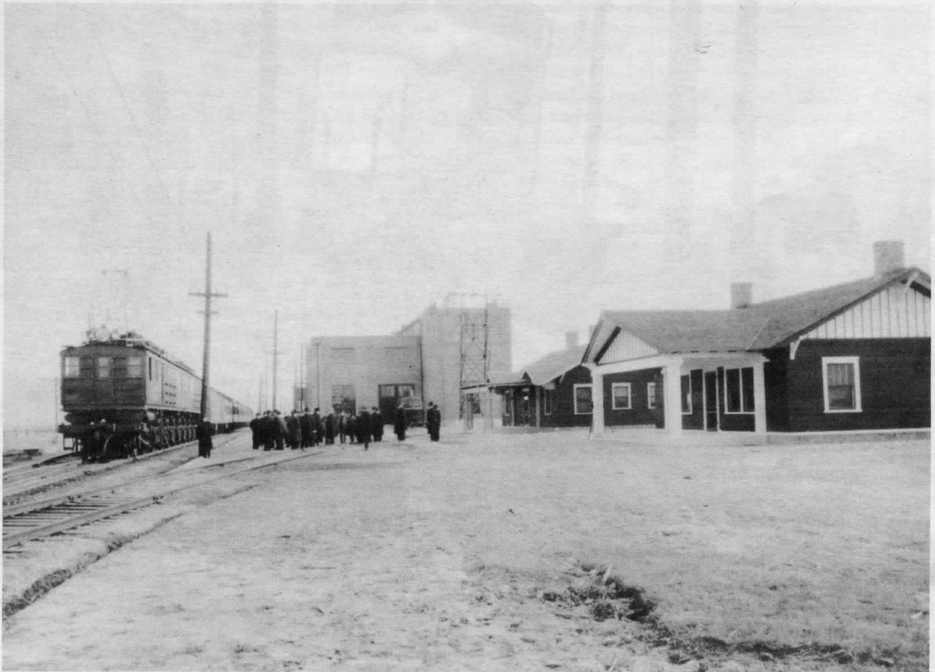
Substation at Piedmont MT. Al Peterson collection
